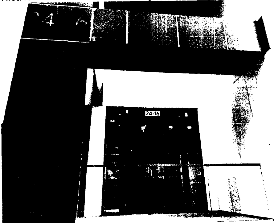
12/5/19 – Detail view of main entrance showing building address
