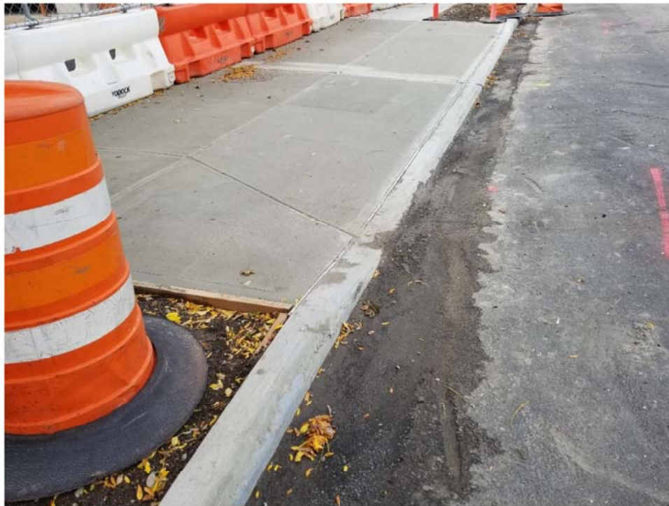
Photo 2 Curb Cut – looking West on Horace Harding Expressway
