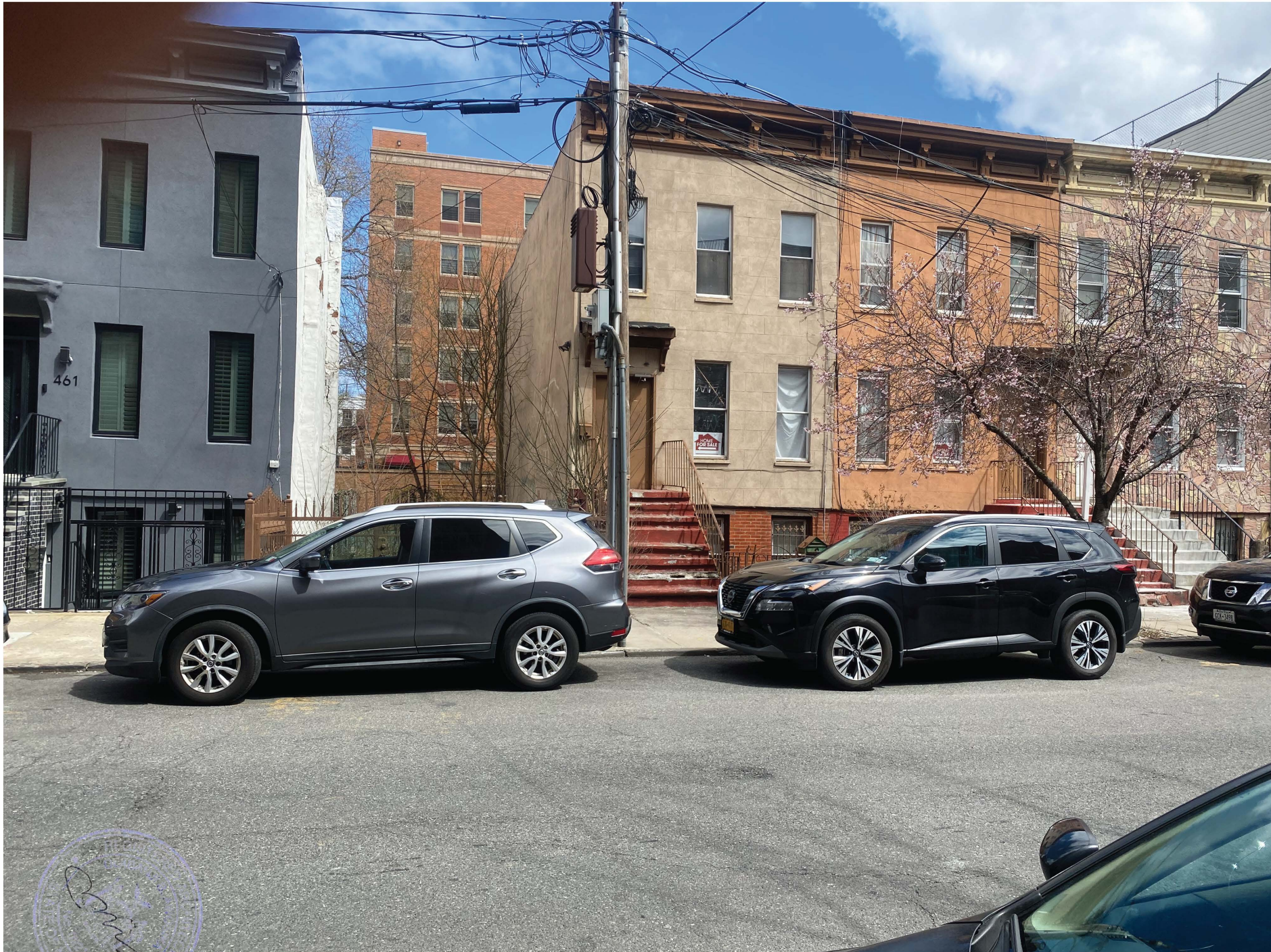
PHOTO FRONT 2 463 EAST 143 STREET, BRONX
