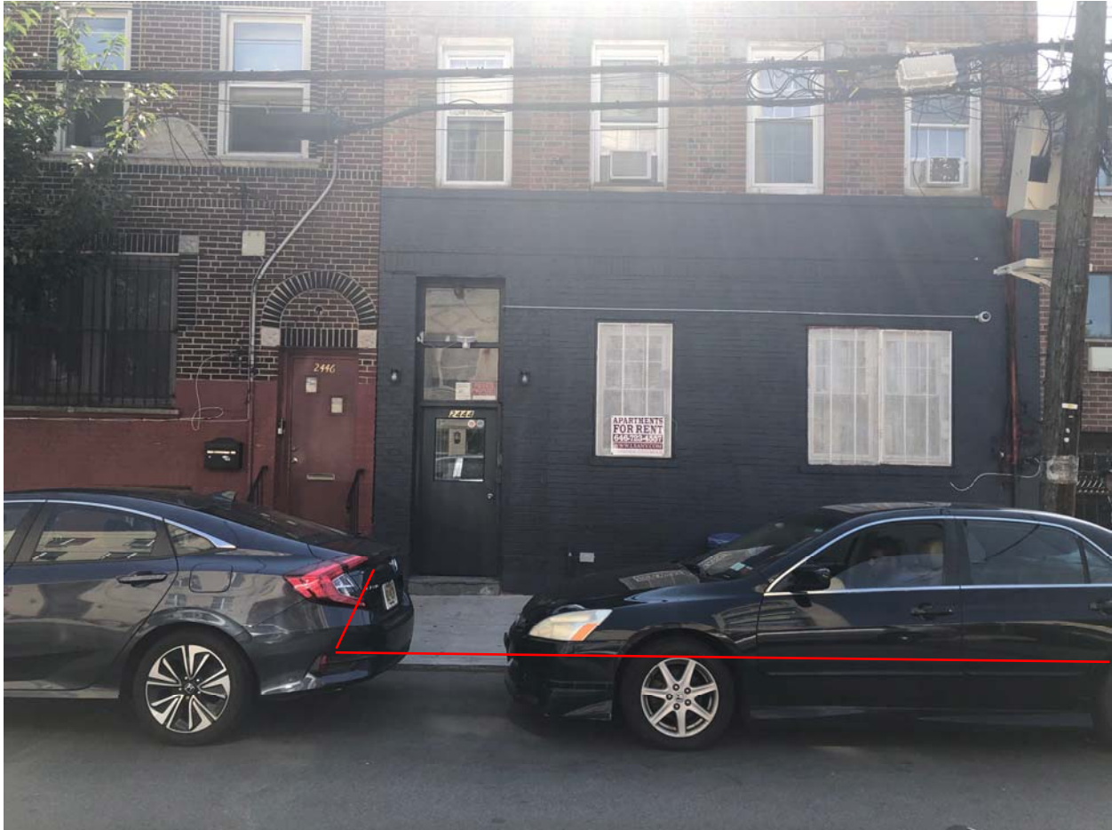
CAMBRELENG AVE FRONT VIEW
