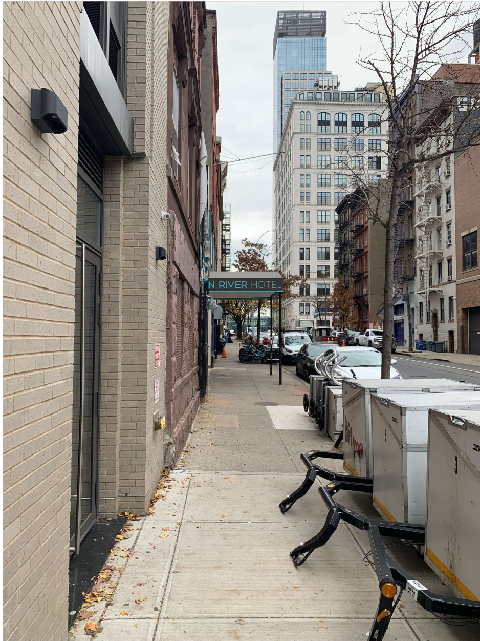
RIGHT SIDE OF 440 WEST 36 th Street Manhattan NY 10018
