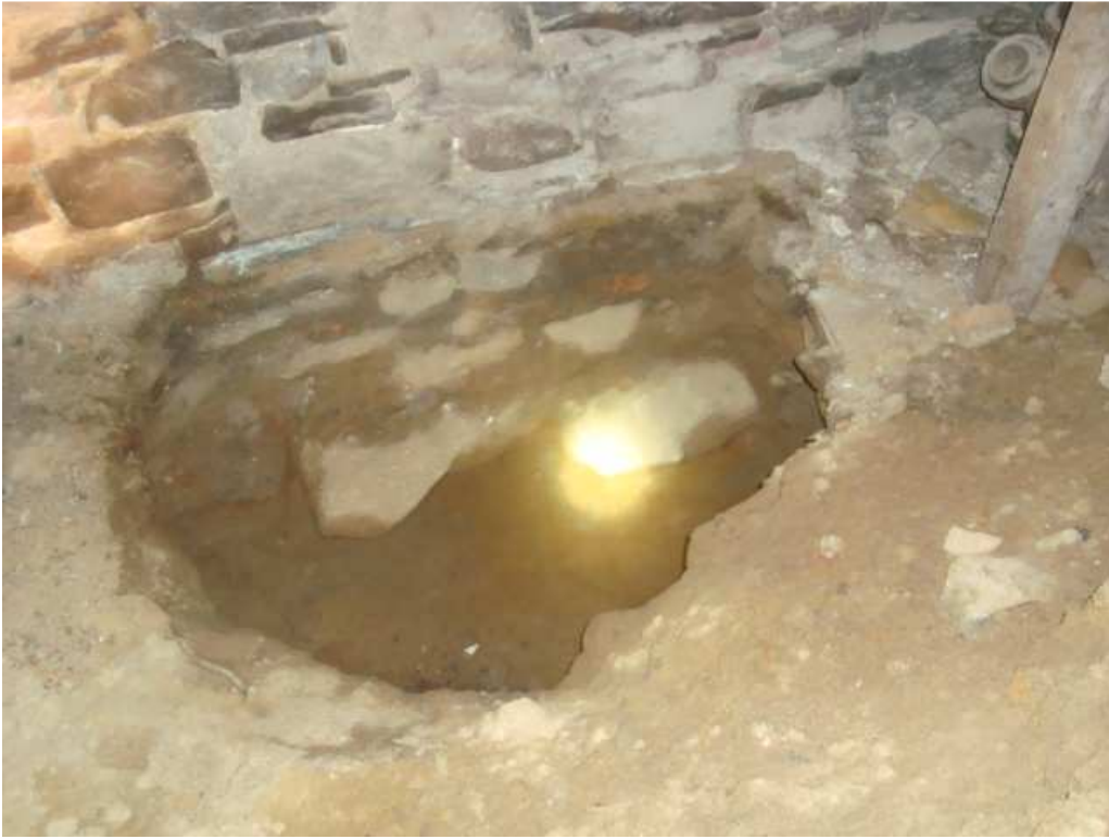
TP3 – West wall center
