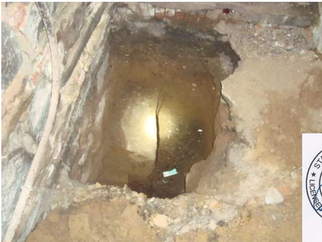
TP2 – Southeast corner
